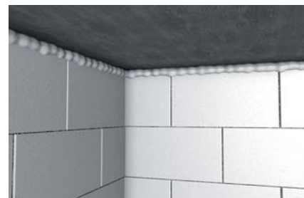
Closing joints in structural work
