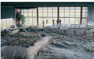
In 1985, the suspended concrete ceiling of an indoor swimming pool collapsed in Uster, Switzerland. The stainless steel ceiling attachments exhibited no external defects, but were completely destroyed internally in some cases due to stress corrosion cracking.
