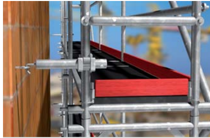
Scaffold anchoring
