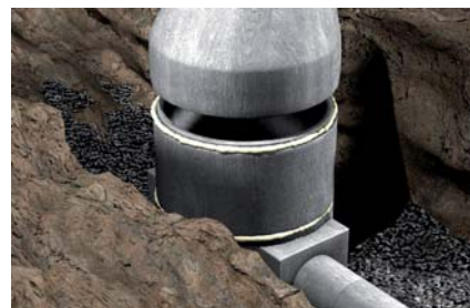
Sealing concrete manhole rings
